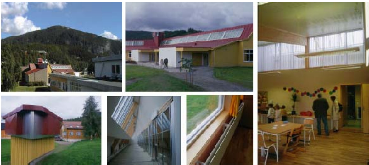
Figure 16 The Media School in Grong, Norway: an example of stack- and wind-assisted mechanical ventilation
