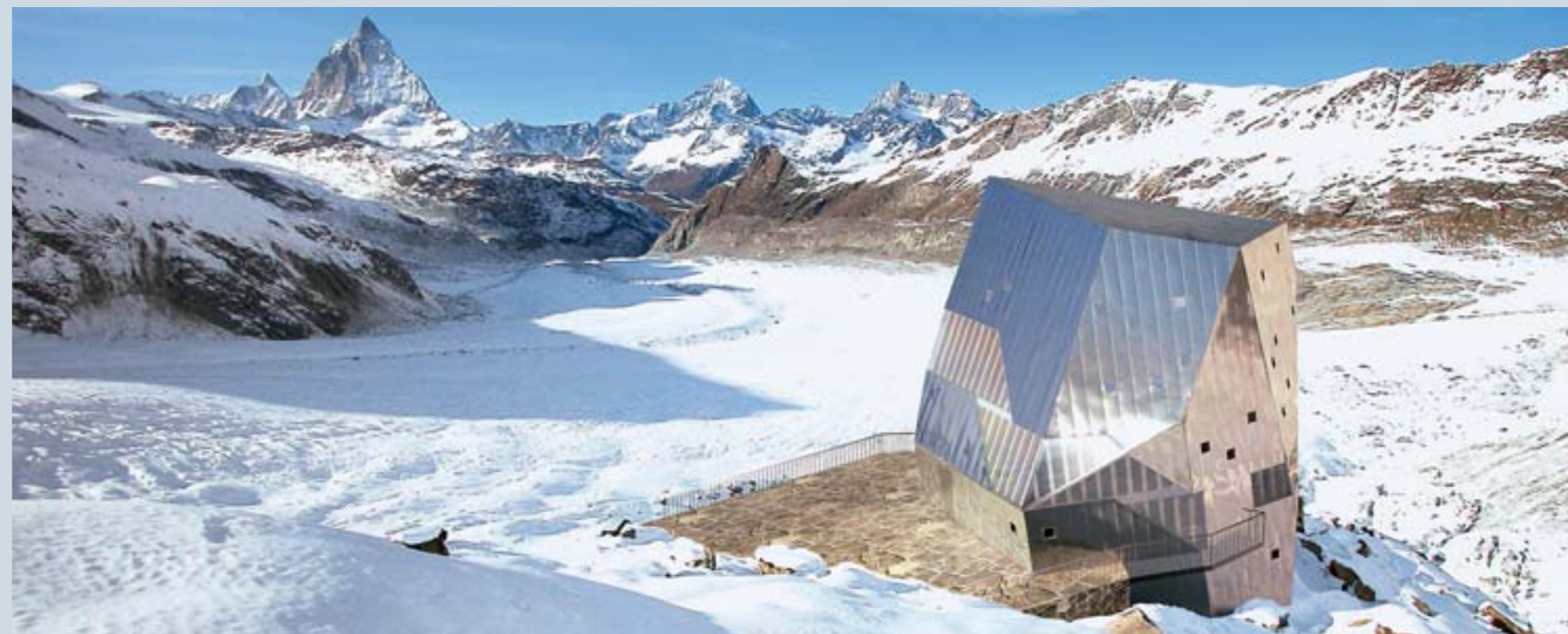
Weather predictions and building automation will be tested in a pilot facility at 2,795 meters. Siemens researcher Dr. Jürg Tödli (photo below) and partners are key players in the project.
