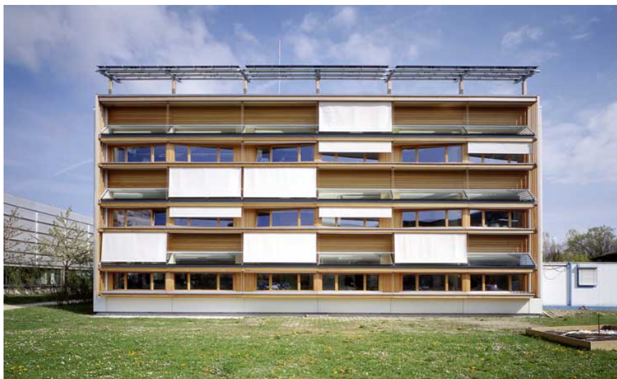
Figure 8.8: The LESO experimental building on the campus of EPFL, Switzerland.
