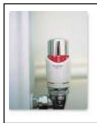
Figure 2. Thermostatic Radiator Valve
